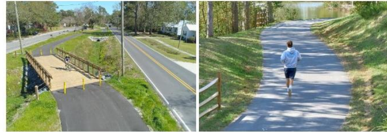
Figure 22. A Trail Next to the Roadway (Left) and a Trail Farther Away from the Existing Road (Right)
